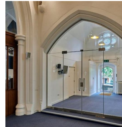
Glazed screen and doors open up views into the church
