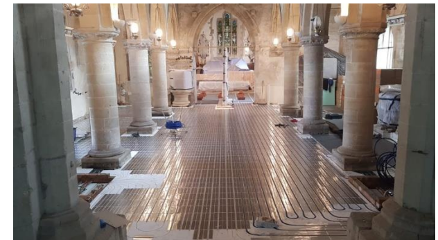
Underfloor heating system being laid within a church
