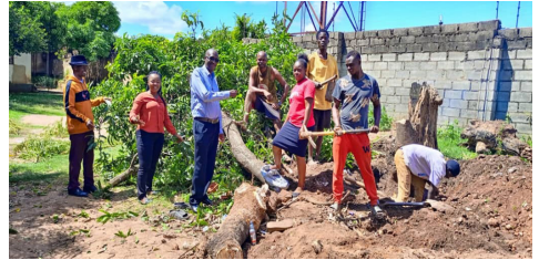
Members of St Paul's, Chipata South laying new school foundations.
